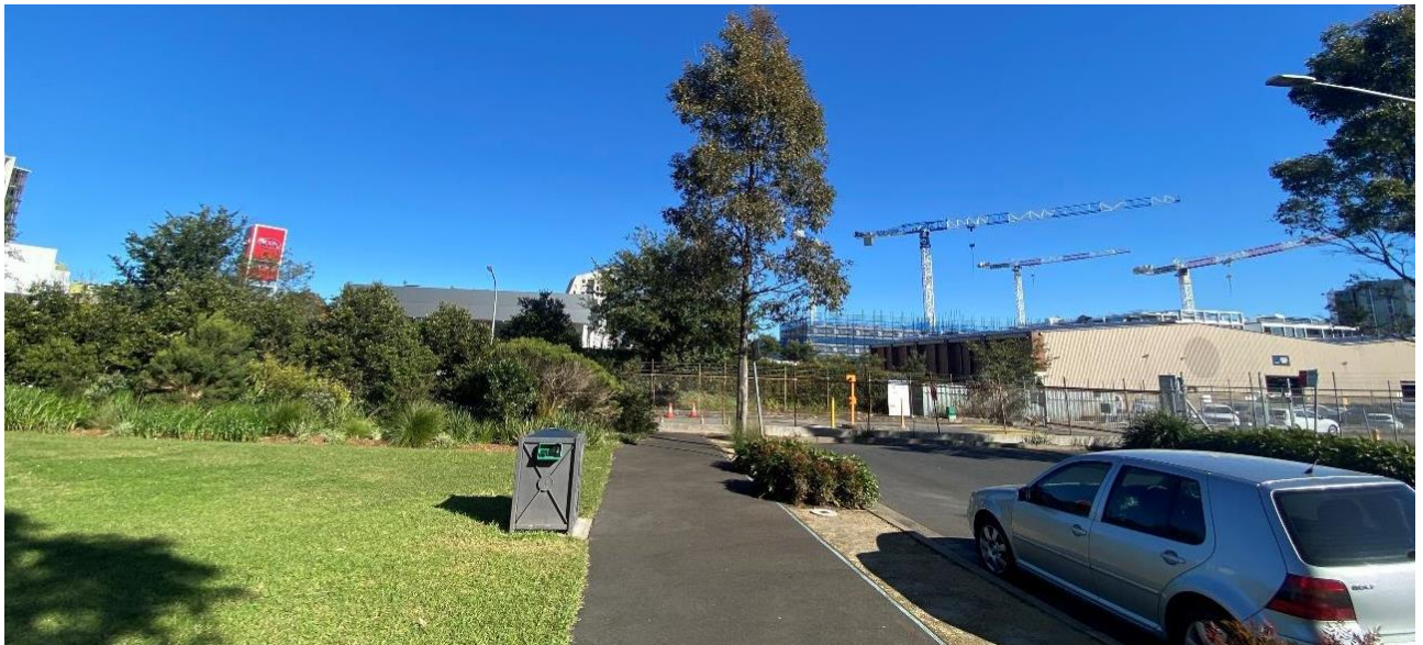
Figure 6 Subject site as viewed from Defries Avenue (Source: Planning Ingenuity)
